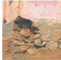
Damage to plinth on south-west corner
