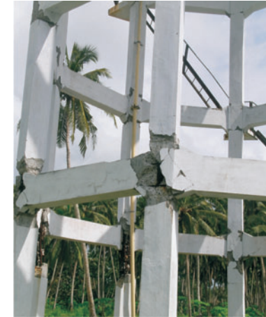
Damage to the village water tank structure
