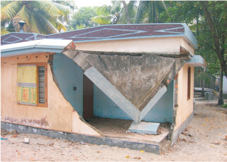
Collapse of north and west walls of the house. Also partial collapse of concrete roof slab
