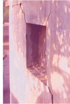
Diagonal cracks near the window on east wall
