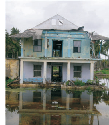
Damage and flooding of the Panchayat building
