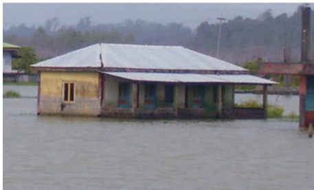
Flooding in the primary school building
