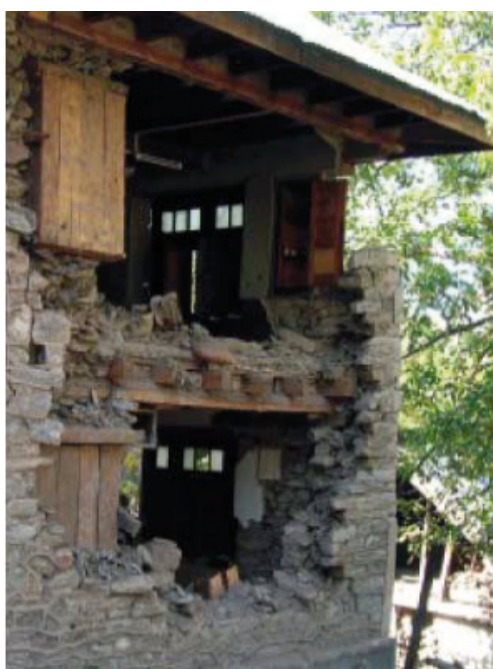
House damage in Kashmir due to the earthquake in 2005
