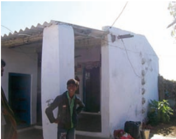
Load-bearing brick masonry with CGI roof
