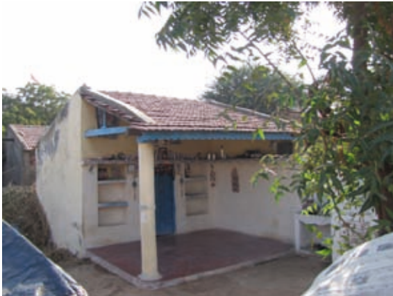
Load-bearing brick masonry with tiled roof
