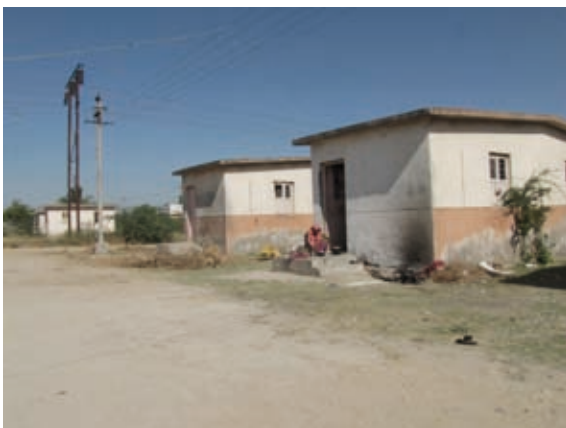
Load-bearing brick masonry with RCC roof
