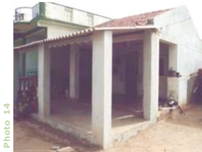
Photo 13-14: New construction along seismic safety norms
