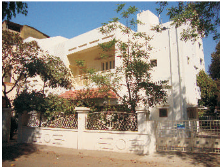
Co-ordinating Office, Ahmedabad
