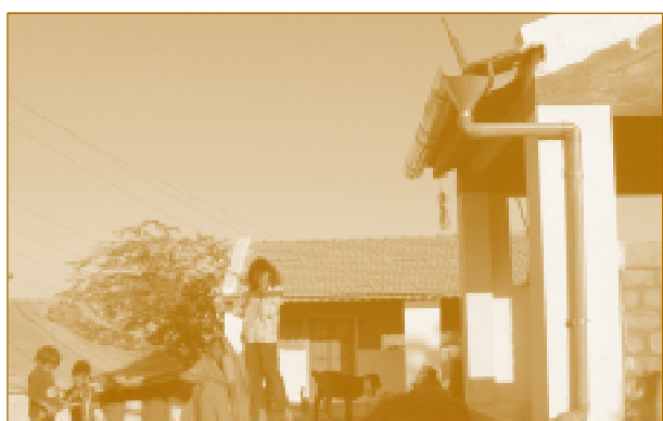
Roof water harvesting, Rabarivas, Bhachau
